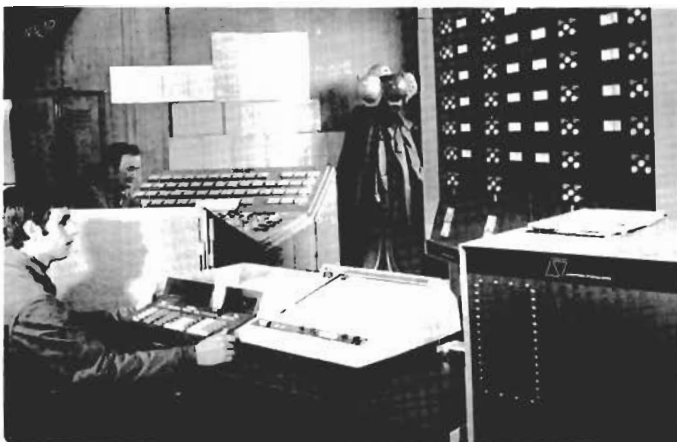
This was the control room for the automatic leveling system. Opposite the 9821 operator is the bank of red and green lights used to signal the frequency, duration, and position of servo activity.
